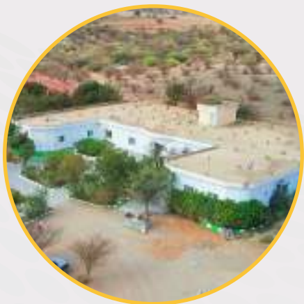
Al Hayat Hospital expansion will begin in 2023 in shaa Allah and will serve the entire region. With the expansion, this hospital will be to provide more essential healthcare services to more and more people in the Horn of Africa.
