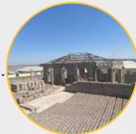
Masjid under construction in Ethiopia - Somali Region.
