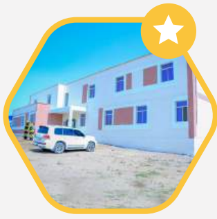
ALHAYATT HOSPITAL EXPANSION
